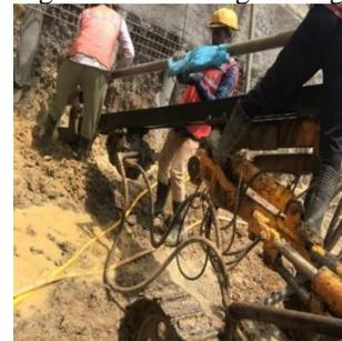
Figure 15: Removing of inserted pipes
