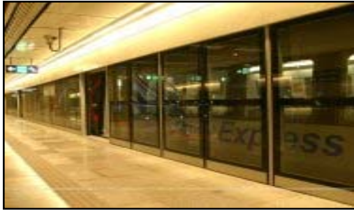
Fig. 3: Platform screened from the tracks
