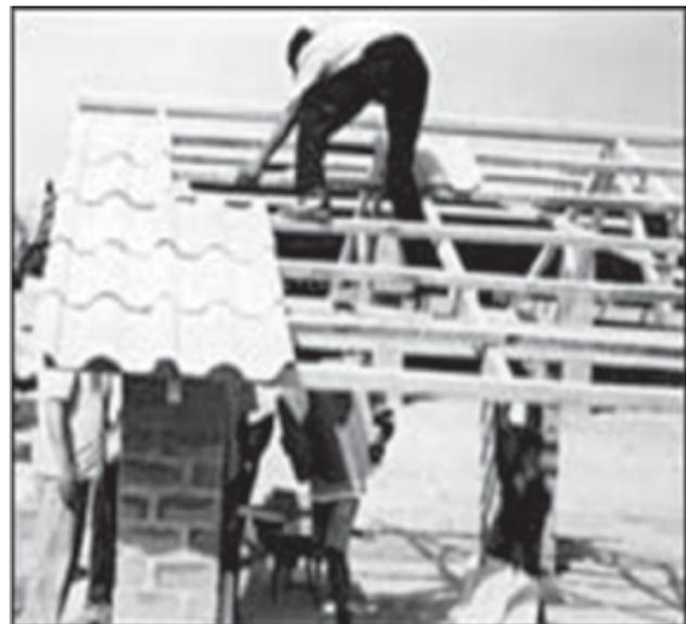
Figure 3. Roof construction using Roman II tiles.
